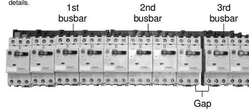
Example of two fork-connection busbars + 3-phase feed-in terminal
